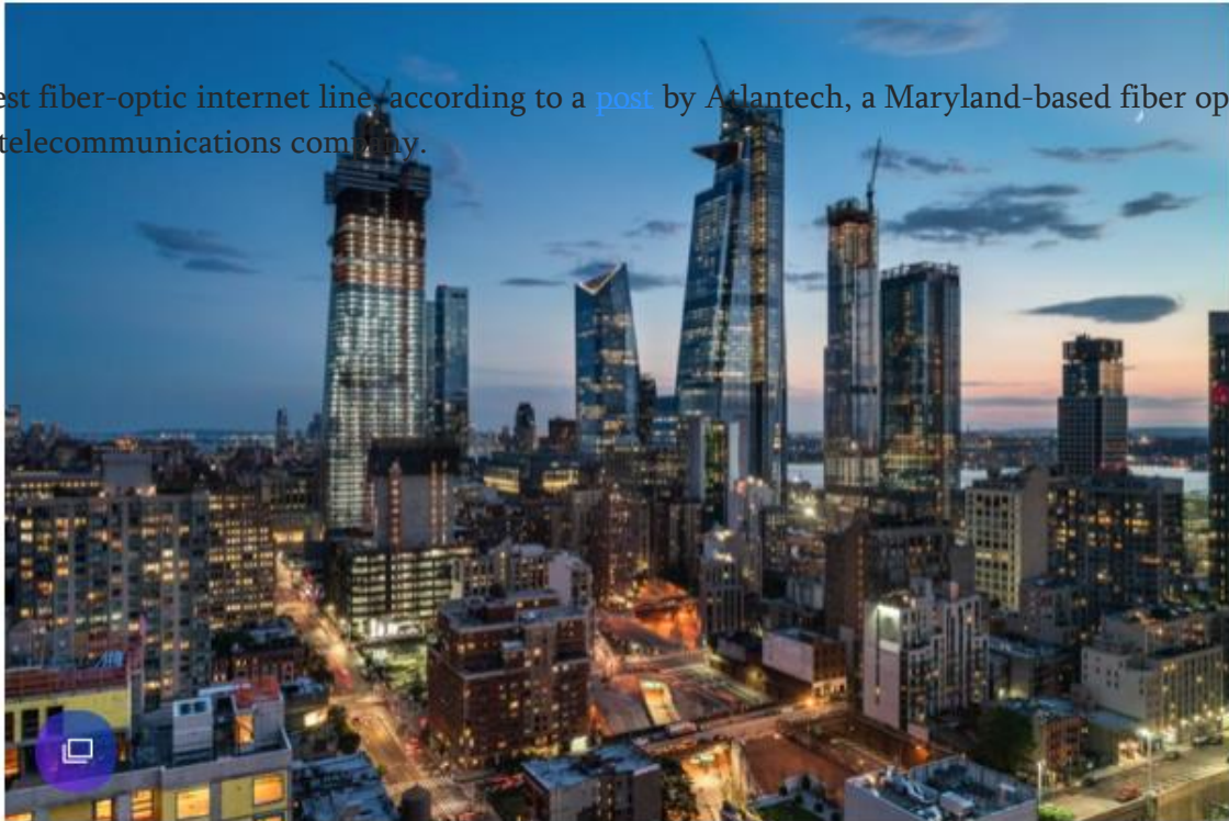
Large scale development projects are underway on the far west side of Manhattan near 34th Street and the Hudson River. This high angle view above Ninth Avenue looks south toward Manhattan West and Hudson Yards, two of the large development projects. Source: Getty Creative.
